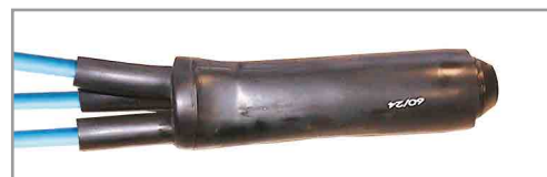
Isolation of cable connection with thermocontracting couplers
